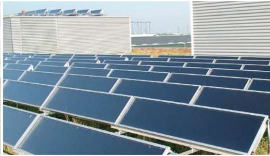
TiNOX is an energy trap. Highly selective blue TiNOX energy absorber coatings take up a lot of energy – some 95% of incident solar radiation – and convert it into heat energy. Conventional absorbers lose a large part of that energy as heat radiation. In contrast, TiNOX energy coatings have an extremely low thermal emissivity of less than 4% in the infrared range to prevent such heat losses. Once the energy has been converted into heat, it stays trapped within the TiNOX absorber.
